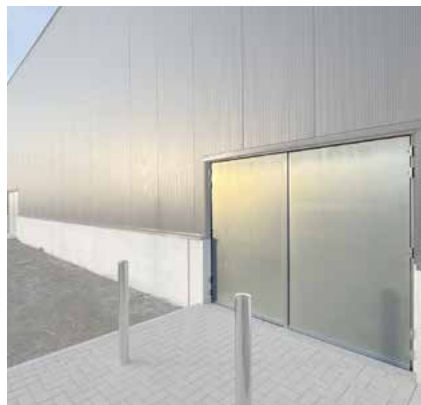
Emergency exit / Exterior
